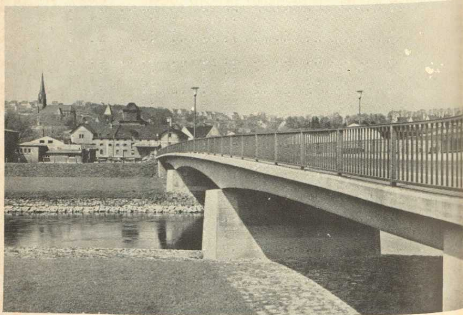
Fröndenberg: Neue Ruhrbrücke
